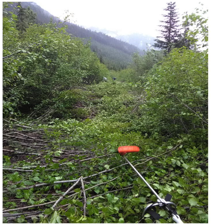
Alder enclosed trail being cleared with 1-power trimmer and 2 crew removing cuttings.
