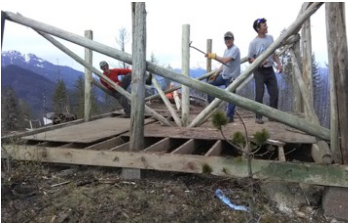
Salvaged materials were carefully stacked for use on the
