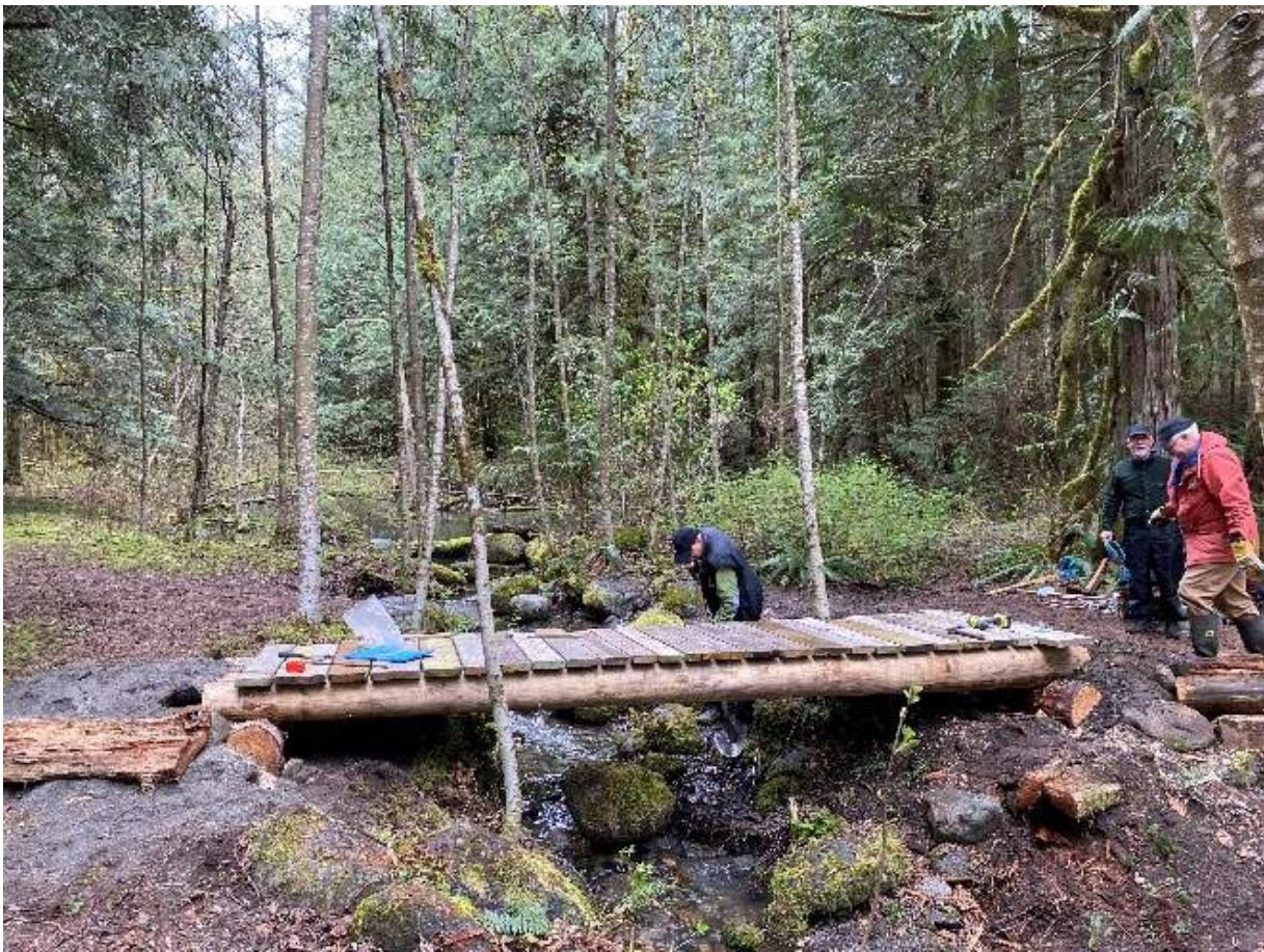
The third bridge shown below was constructed using firm tree stringers from Wayne Furnass and a bridge deck that was salvaged from a nearby dry stream bed where it appeared to have been deposited during the November floods.
