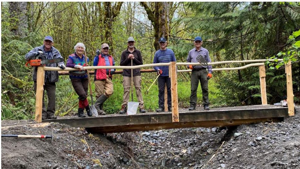
Erosion of the trail near the fishermen's dike by Slesse Creek required reconstruction of a section of the trail; new TCT signage and reggrading was complete.
