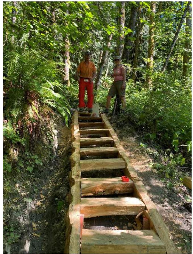
A new bridge was constructed at the mid point of the Tolmie section using a cedar tree for the stringers and decking cut from first growth stumps in the area.
