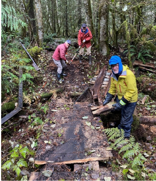
The curbs were added and the edge of the decking were trimmed.
