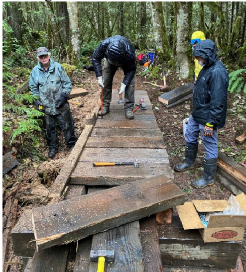
The curbs were added and the edge of the decking were trimmed.
