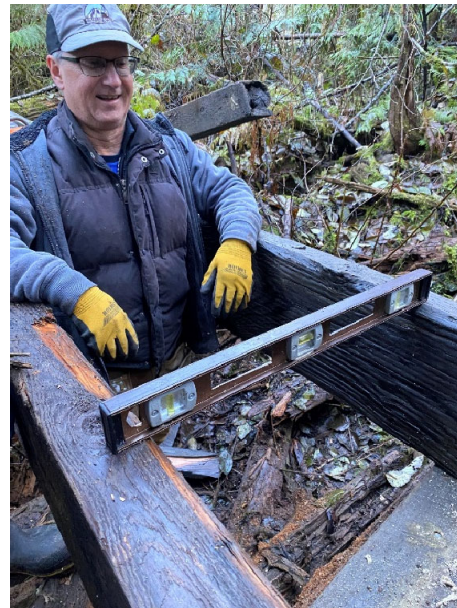
The level of the stringers was confirmed.
