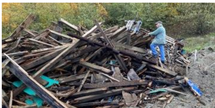
Jim S examines the pile of material at Centre Creek pit to identify useable timbers.
