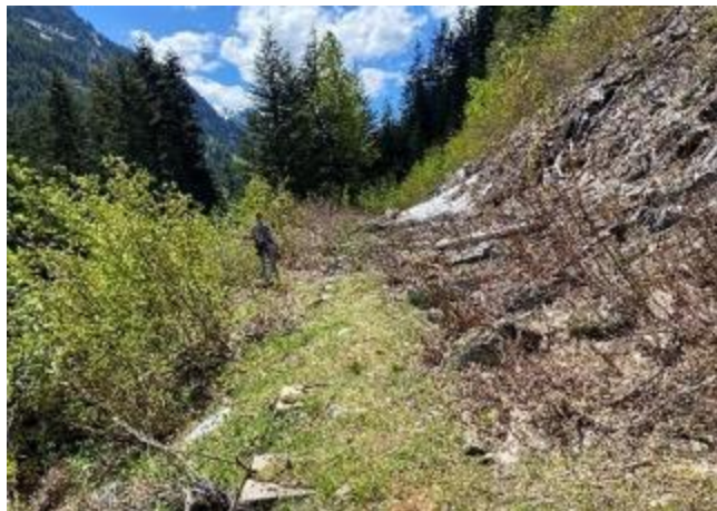
Remnants of a wooden snow shed and concrete footings.
