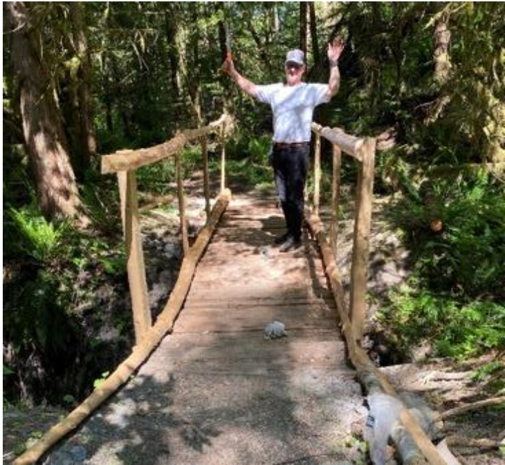
Railings were added to the log bridge on the Tolmie Section and curbs were added to 4 bridges in Thurston Meadows.
