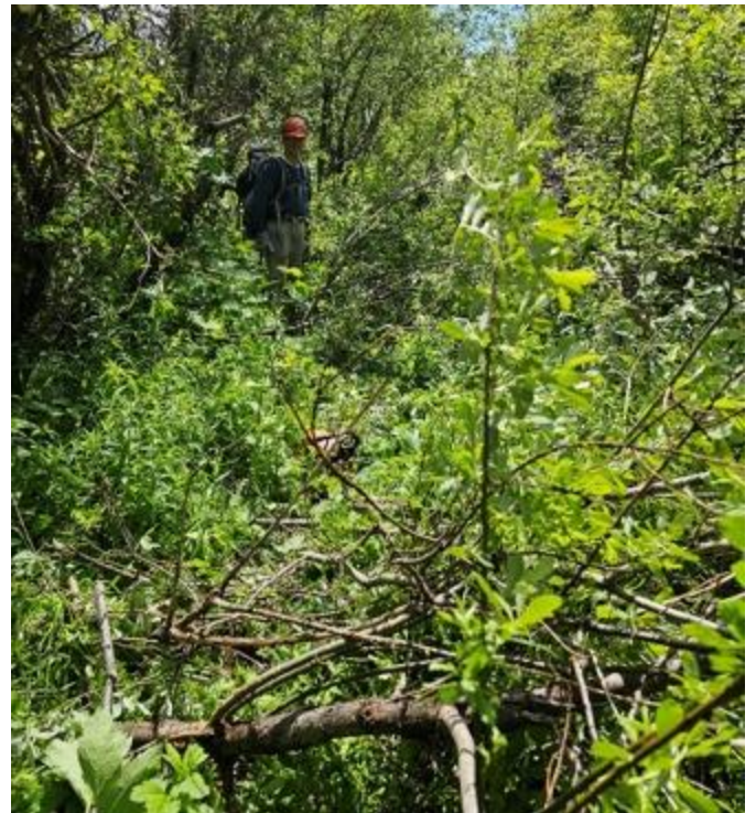
The chainsaw, power trimmers and loppers were used to clear the encroaching brush of "the green wall" as Rob calls it. Before clearing.
