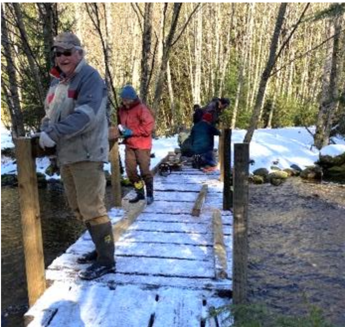
Temporary approach ramps at each end of the bridge were added.
