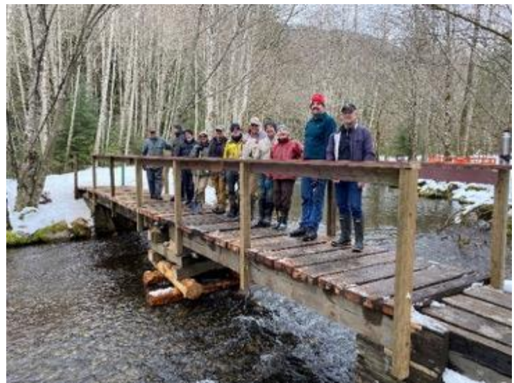
The railings were completed with lumber obtained from a local small sawmill and purchased by Trails BC.
