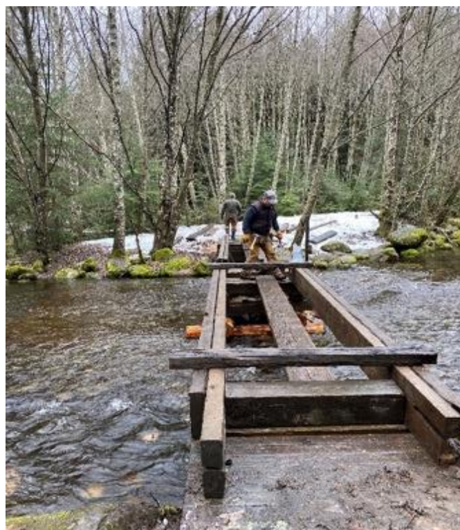
Next we cut and placed the decking.
