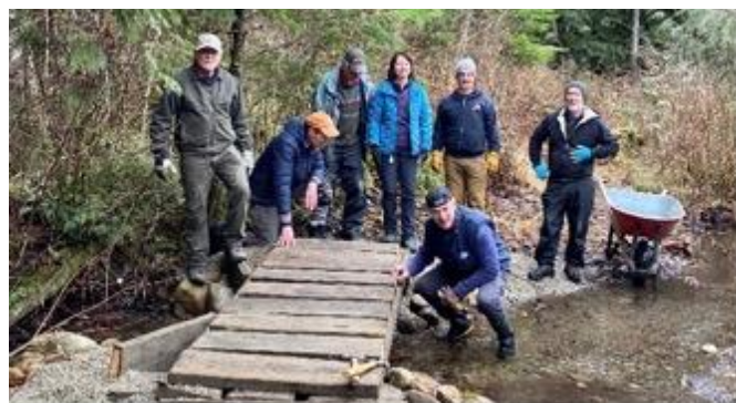
Next we cut and placed the decking.
